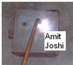
Final preheating before pouring
